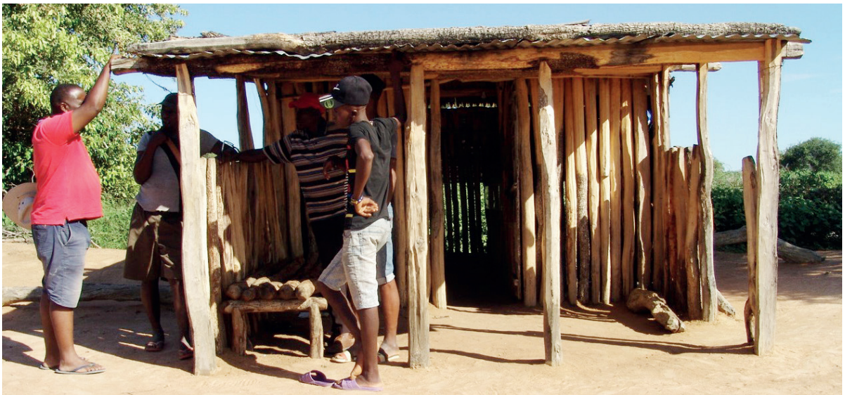
Figure 43: Examples of buildings constructed with corrugated a) iron/zinc, b) stick and mud and c) wood
