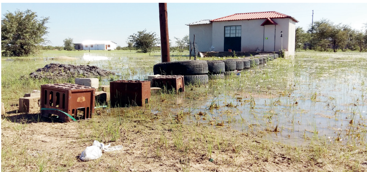
Figure 30: An example of modification of the surroundings to cope with flooding. In this case, old tyres and crates were used to facilitate access to the buildings during the flooding. The effectiveness of this rudimentary modification in the case of extreme floods is not known.
