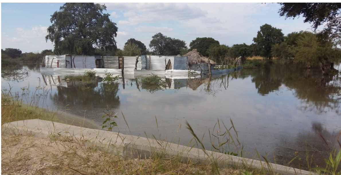
Figure 108: An example of a house faced with multi-hazards. In this case, the house is flooded and at the same time rooms are built with corrugated iron/zinc materials which expose inhabitants to heatwave.
