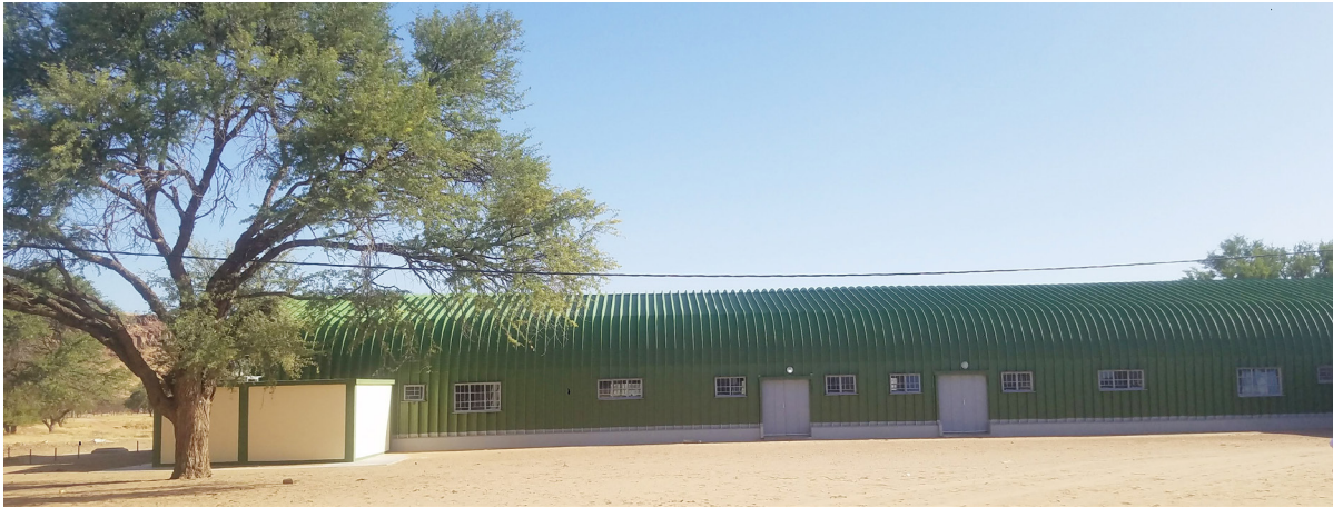
Figure 71: An earthquake-resistant hostel block constructed recently in Anker for Edward //Garoeb Primary School, Kunene Region
